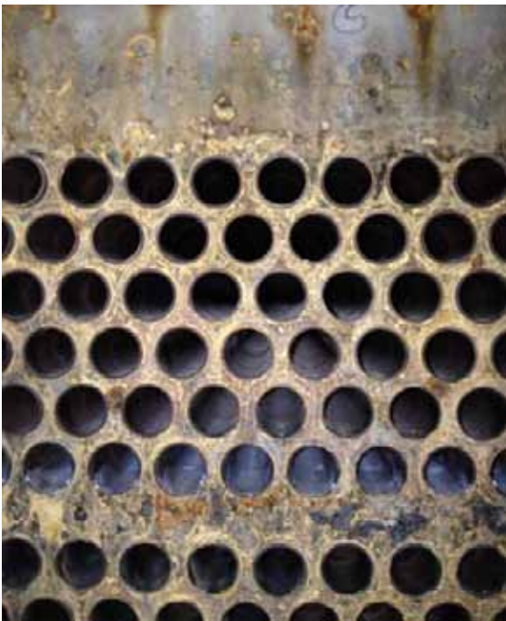
No scale formation after using Vulcan
